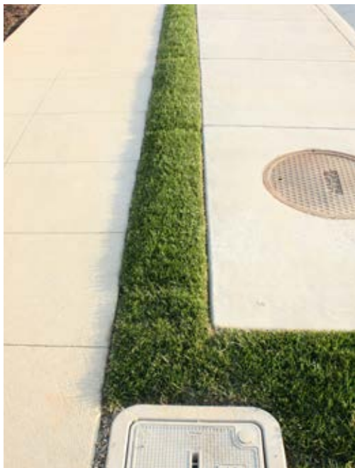
Narrow strips or next to roadways
