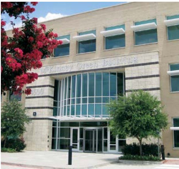
Eliminate overspray on buildings
